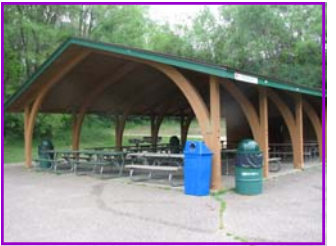
FOR Parks Shelter
