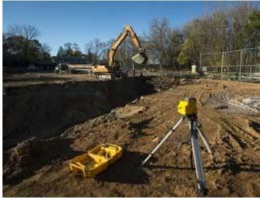
Rainwater will be collected, filtered and used to water playing fields at Upper Villa Park in Roseville. Construction started this month.
