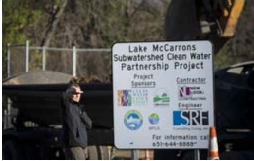
Roseville Parks and Recreation Director Lonnie Brokke looked over the construction site at Upper Villa Park.
