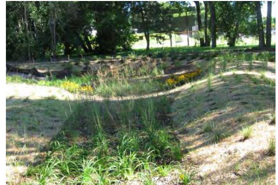
Aladdin Street Bioinfiltration Basin Retrofit (Photo Source: Ramsey Conservation District)
