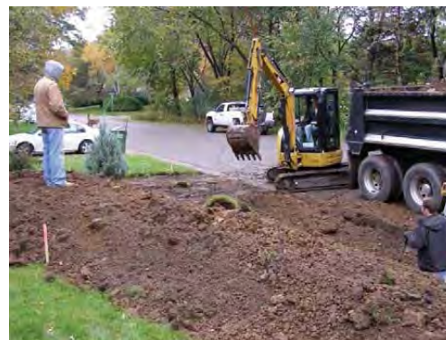
Rain garden being constructed in Rosewood Neighborhood
