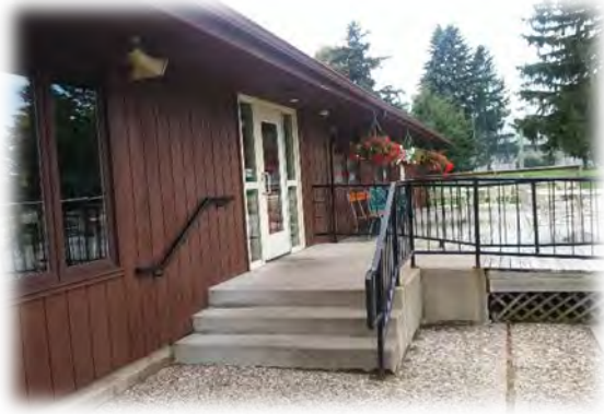
Clubhouse entrance from the parking lot
