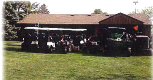
Cedarholm maintenance facility & storage
