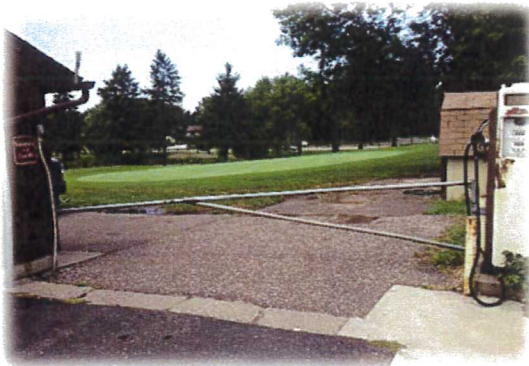
Cedarholm maintenance support area
