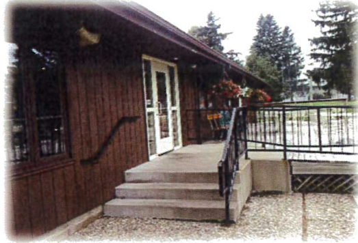
Clubhouse entrance from the parking lot
