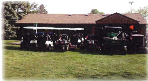
Cedarholm maintenance facility & storage
