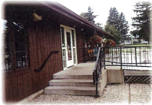
Clubhouse entrance from the parking lot
