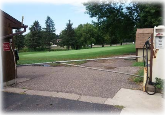
Cedarholm maintenance support area
