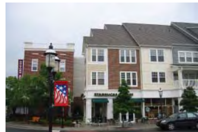
Window and door openings
