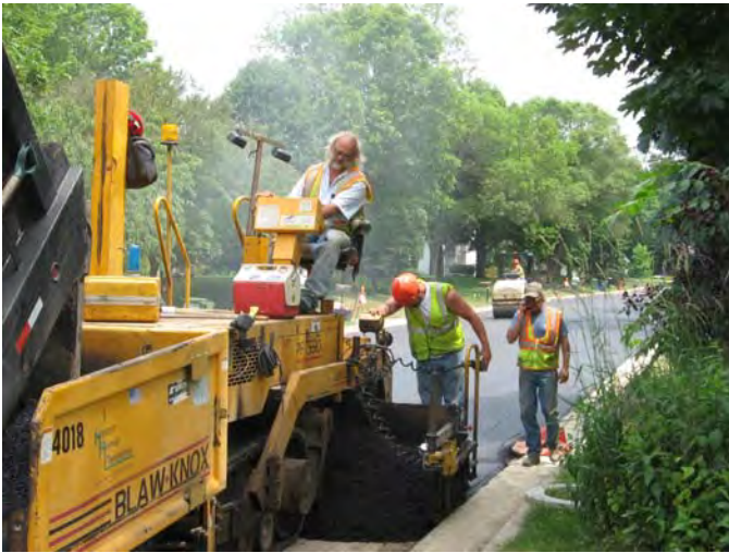
Bituminous paving on Lydia Drive
