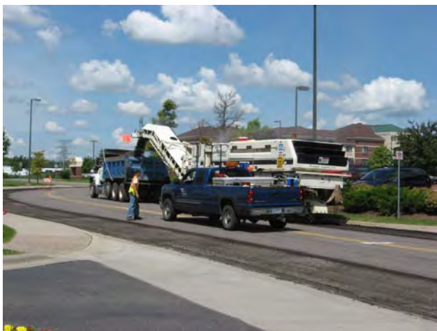
Milling of existing pavement on Centre Pointe Dr.
