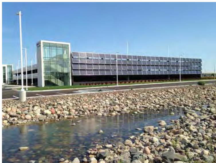
Metro Transit's Hwy. 610 & Noble Parkway Park & Ride has an array of solar panels to power lighting in the ramp. The Council uses “behind-the-meter” solar power at some of its facilities, and now has three procurements in process for community solar gardens.
