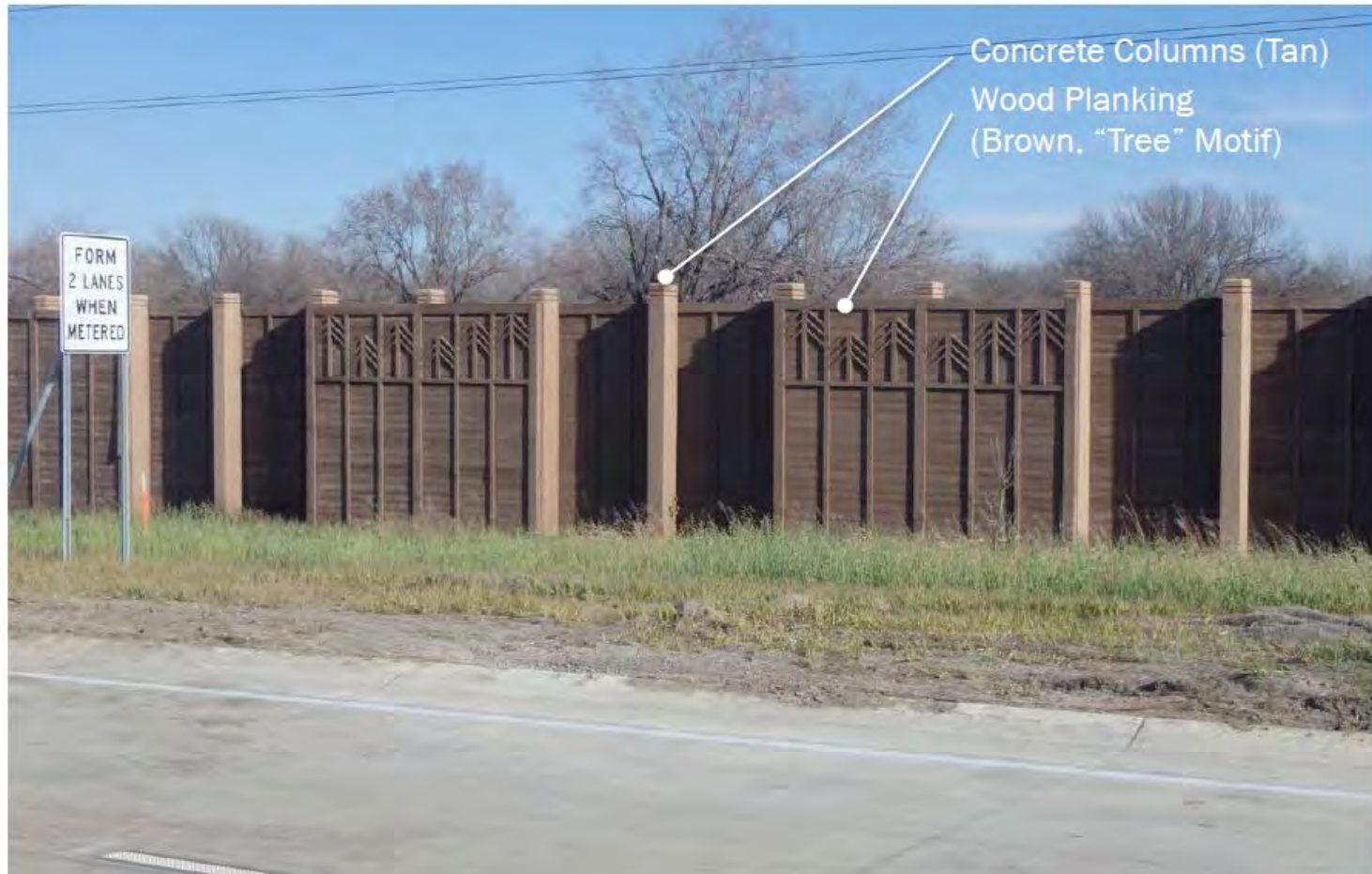
► Noise Walls at CR 96 Interchange
