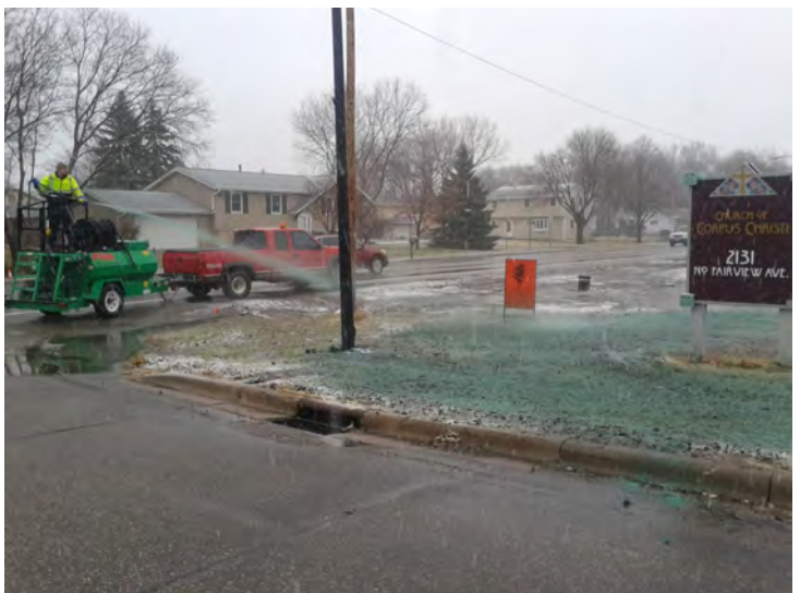
Above: The contractor hydromulching in the snow. Proof that it can be done.
