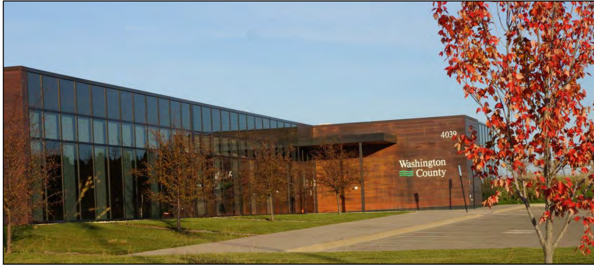
Existing facility, Washington County Environmental Center, MN
