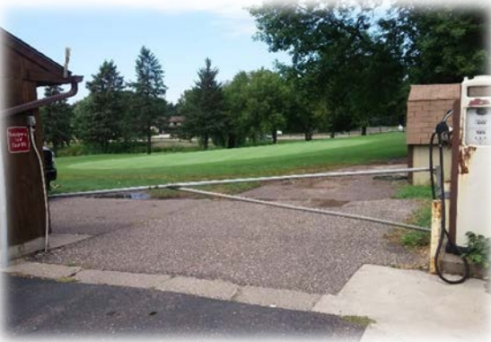
Cedarholm maintenance support area
