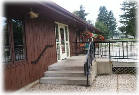
Clubhouse entrance from the parking lot
