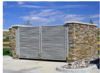
Trash-storage enclosure with masonry walls
