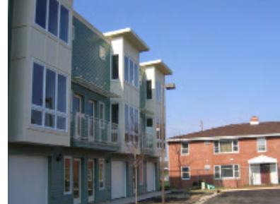
Tuck-under garages take access from rear of building
