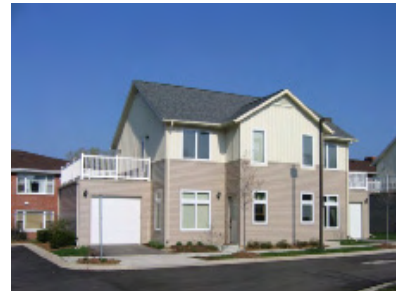
Attached garage doors occupy less than 50% of building front
