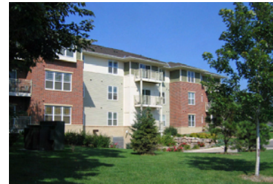
Building with street-facing façade articulated by offsets, changes in materials, and window placement
