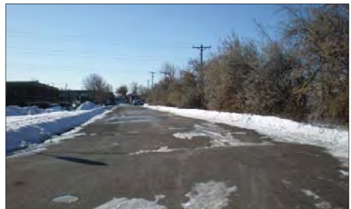
Prior Avenue. Reconstruction of this street will benefit new and existing development.
