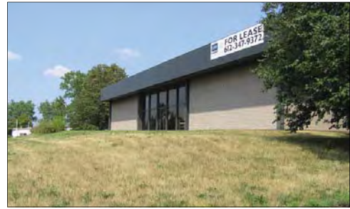
The future entrance of Twin Lakes Parkway from I-35W and Cleveland Avenue.
