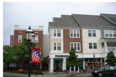
Window and door openings.
